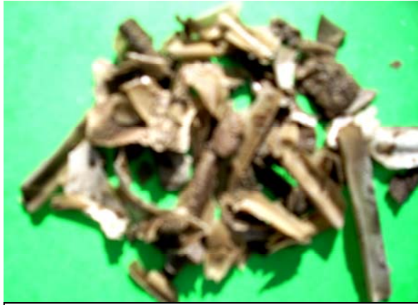
Scale from NCD Treated Cooling Tower
