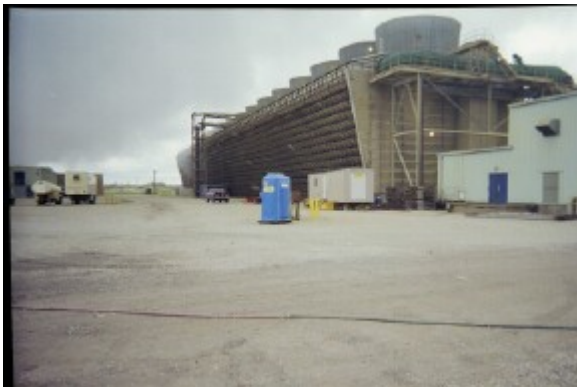
Unit 4 Cooling Tower
